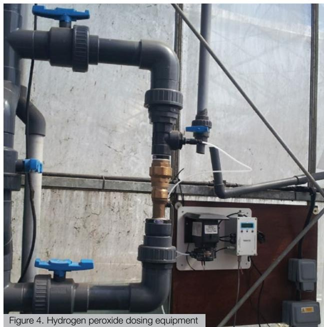
Figure 4. Hydrogen peroxide dosing equipment
