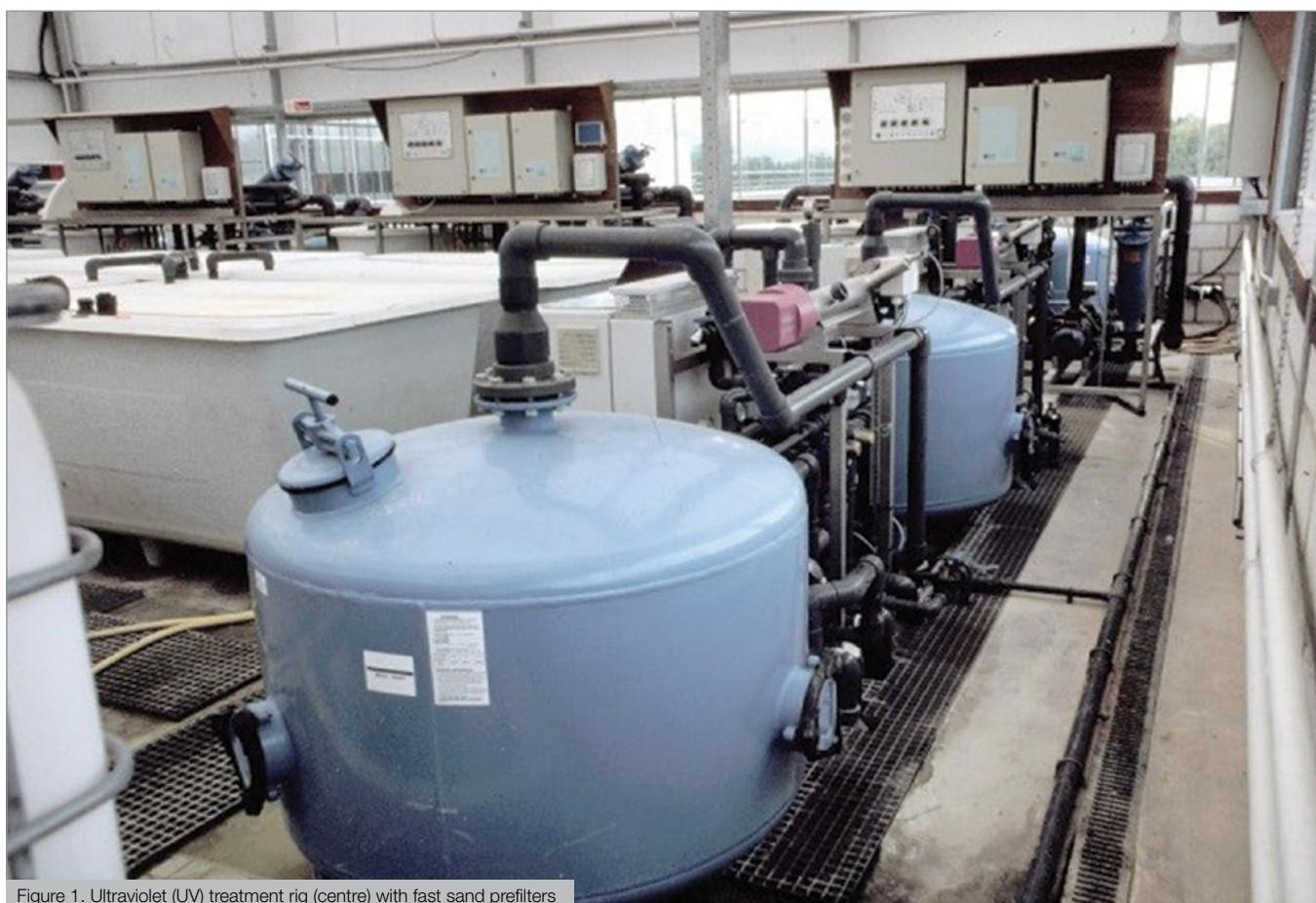
Figure 1. Ultraviolet (UV) treatment rig (centre) with fast sand prefilters
